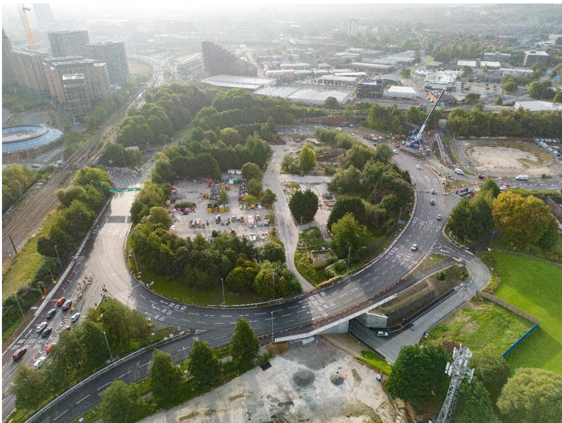
Aerial view of the gyratory, looking south, with the crane used in the demolition of Spence Lane footbridge in situ
